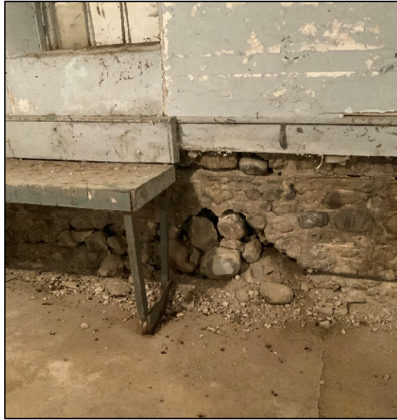
Photograph 5: Destabilized foundation wall, west elevation
