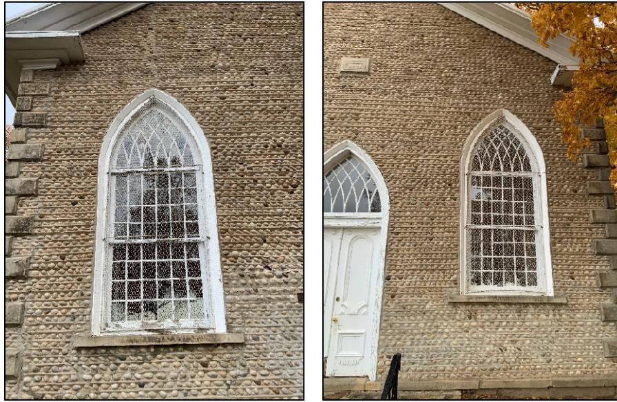
Photograph 13a, 13b: Cracks above front elevation window openings
