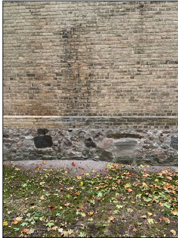
Photograph 7: Mortar deterioration and repairs; rear elevation
