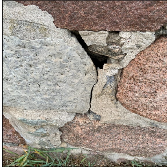
Photograph 9: Failed foundation mortar; evidence of water ingress
