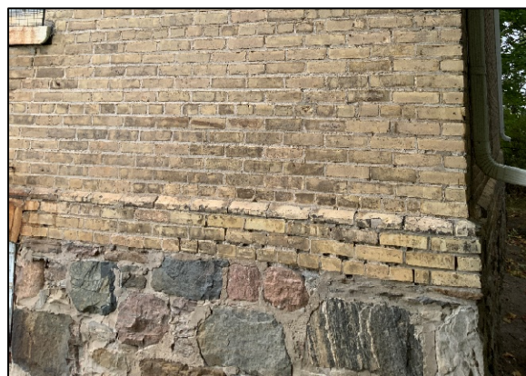
Photograph 8: Mortar deterioration; northeast corner
