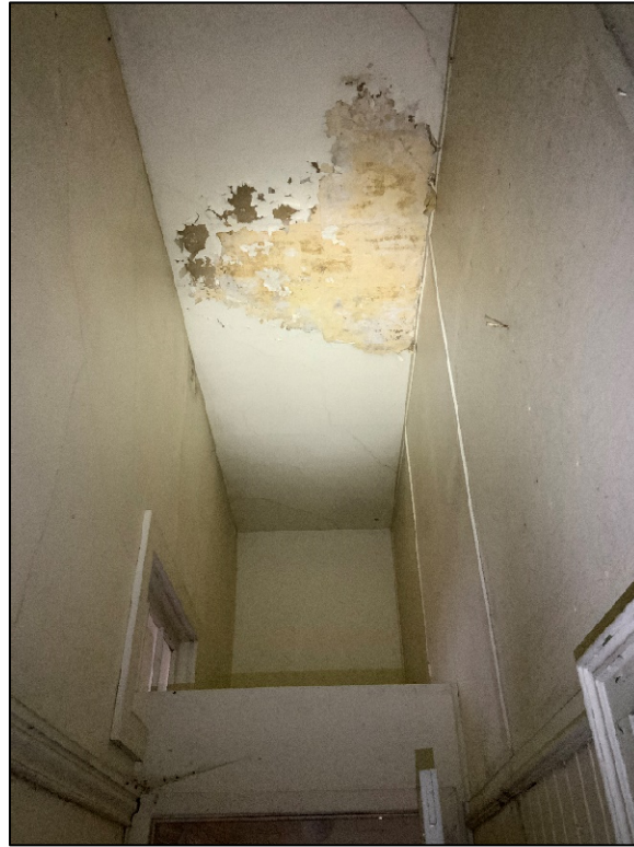
Photograph 2: Water staining on ceiling
