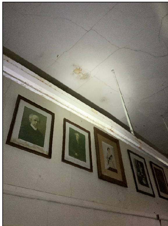
Photograph 1: Cracked plaster finishes in classroom
