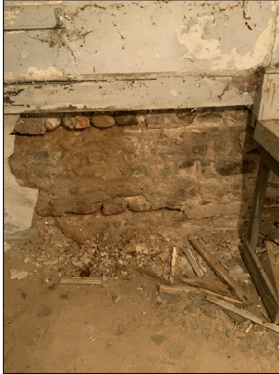
Photograph 4: Exposed foundation wall
